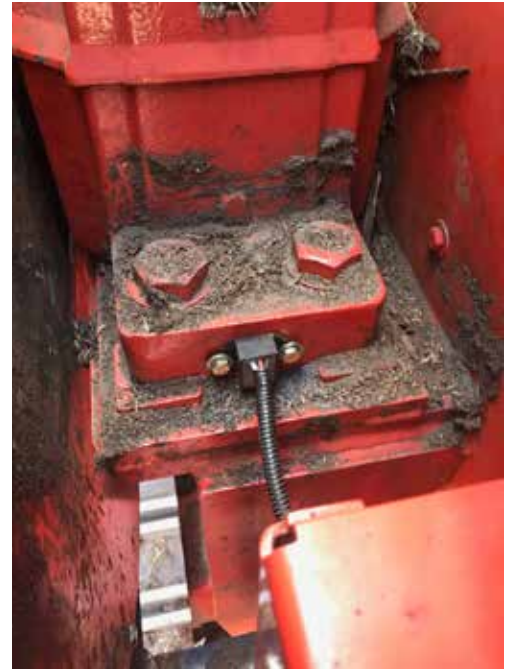
Installed Vtection System
